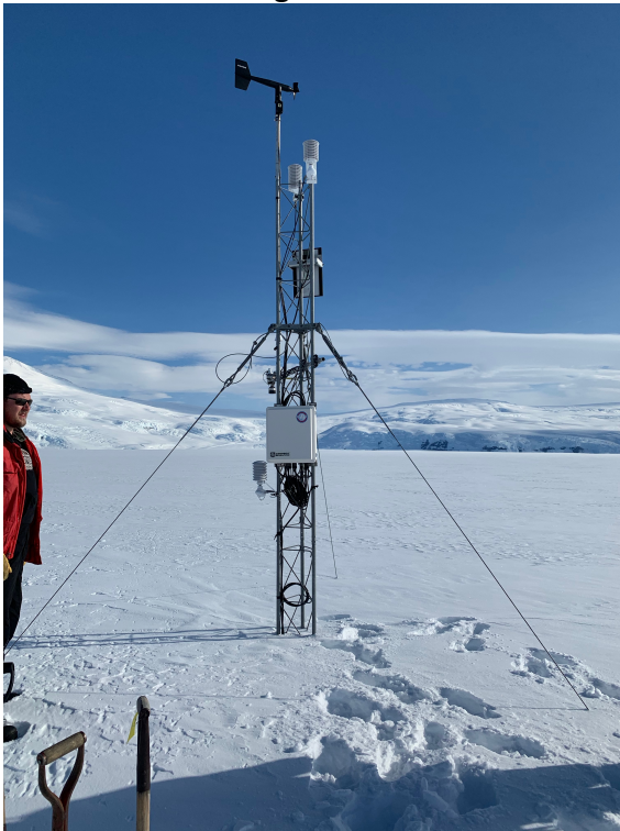
Windless Bight Peripheral port with damage
