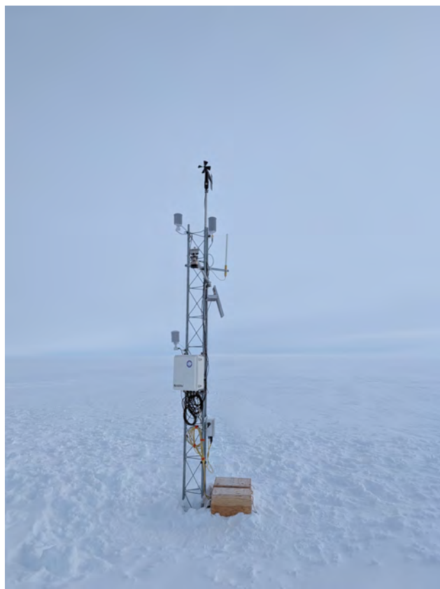
Pointing towards South - After
