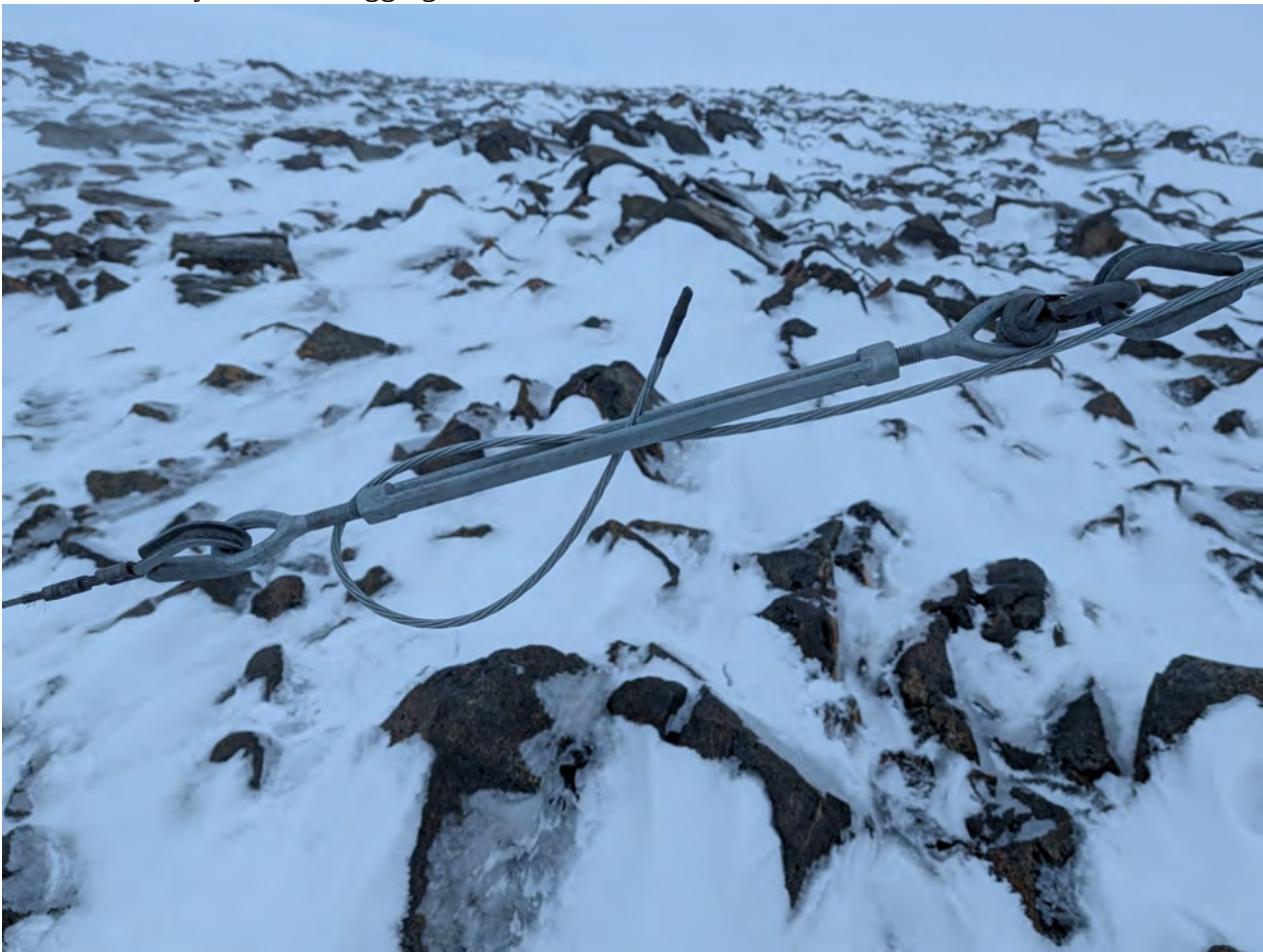
Turnbuckle assembly for tower rigging
