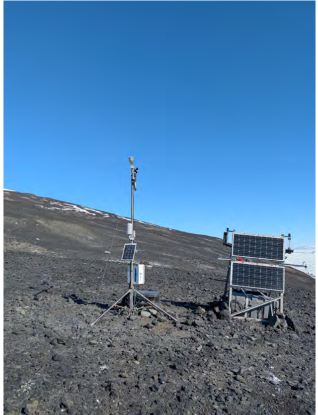
Pointing towards South - After
