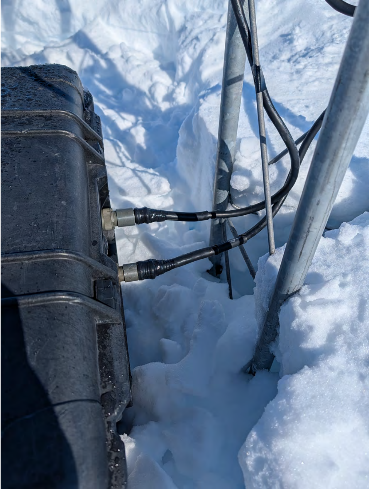
Power system cable strain reliefs - repaired
