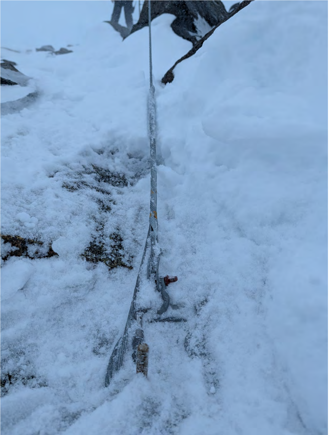
Footing for guy wire drilled into rock
