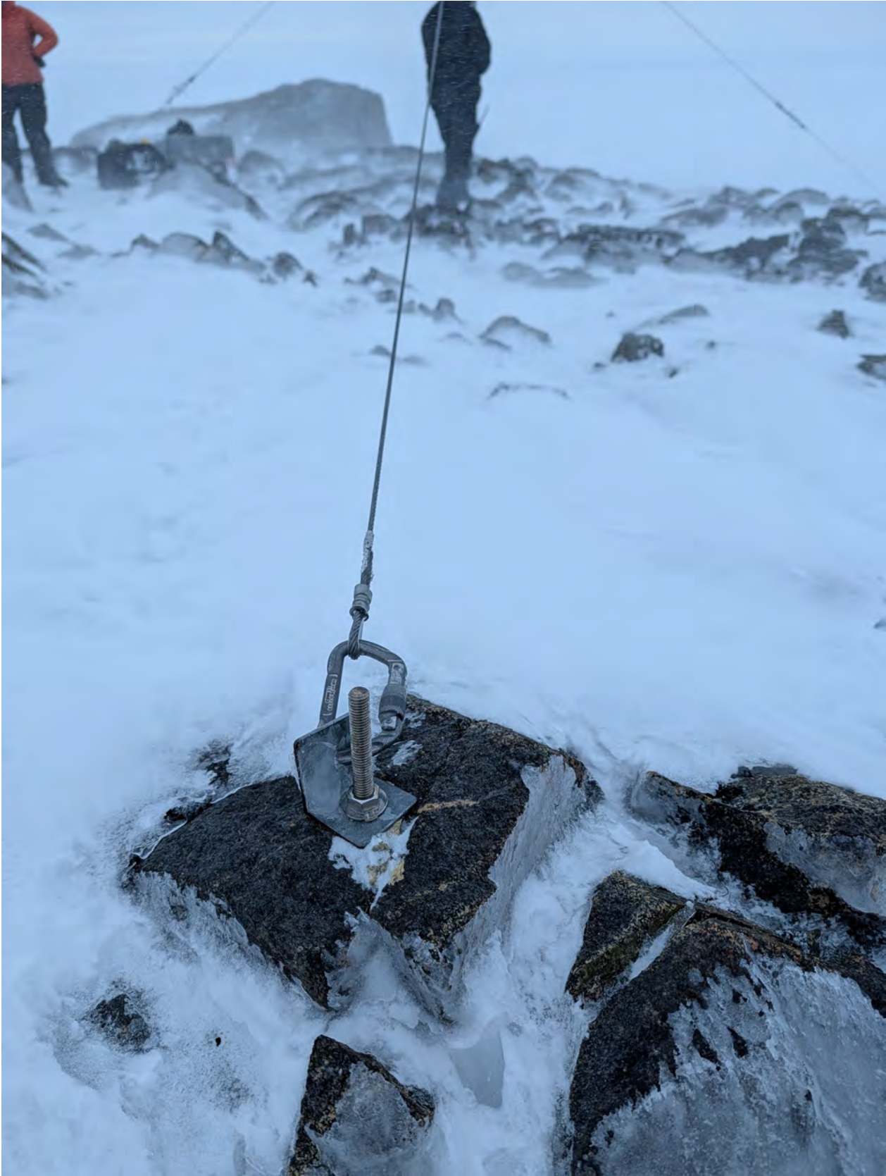
Footing for guy wire drilled into rock
