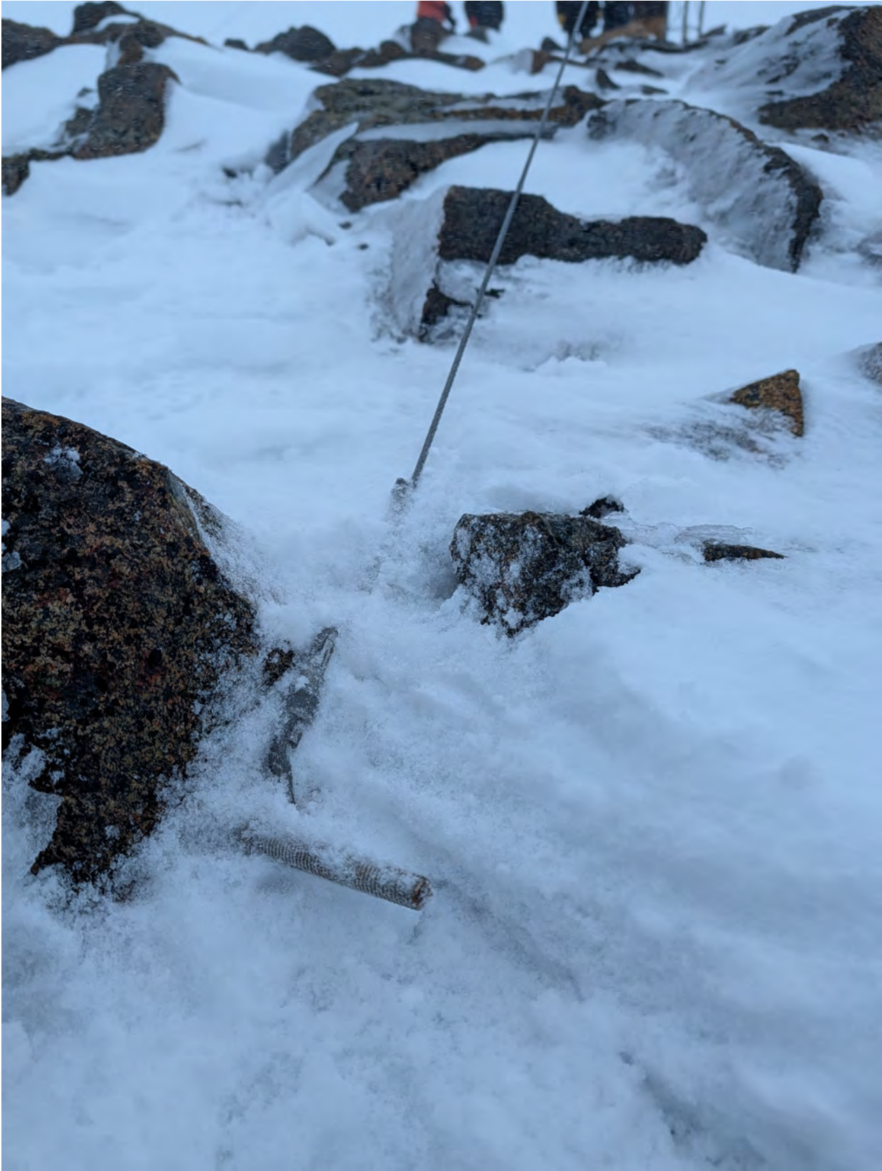
Footing for guy wire drilled into rock
