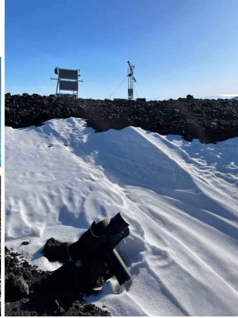
Anemometer on the ground ~30 ft away.
