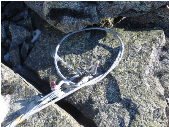
The new guy wire at the anchor.
