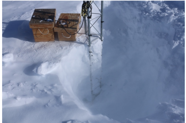
The hole to recover the batteries.
