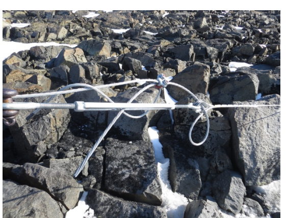
New guy wire at the turnbuckle.
